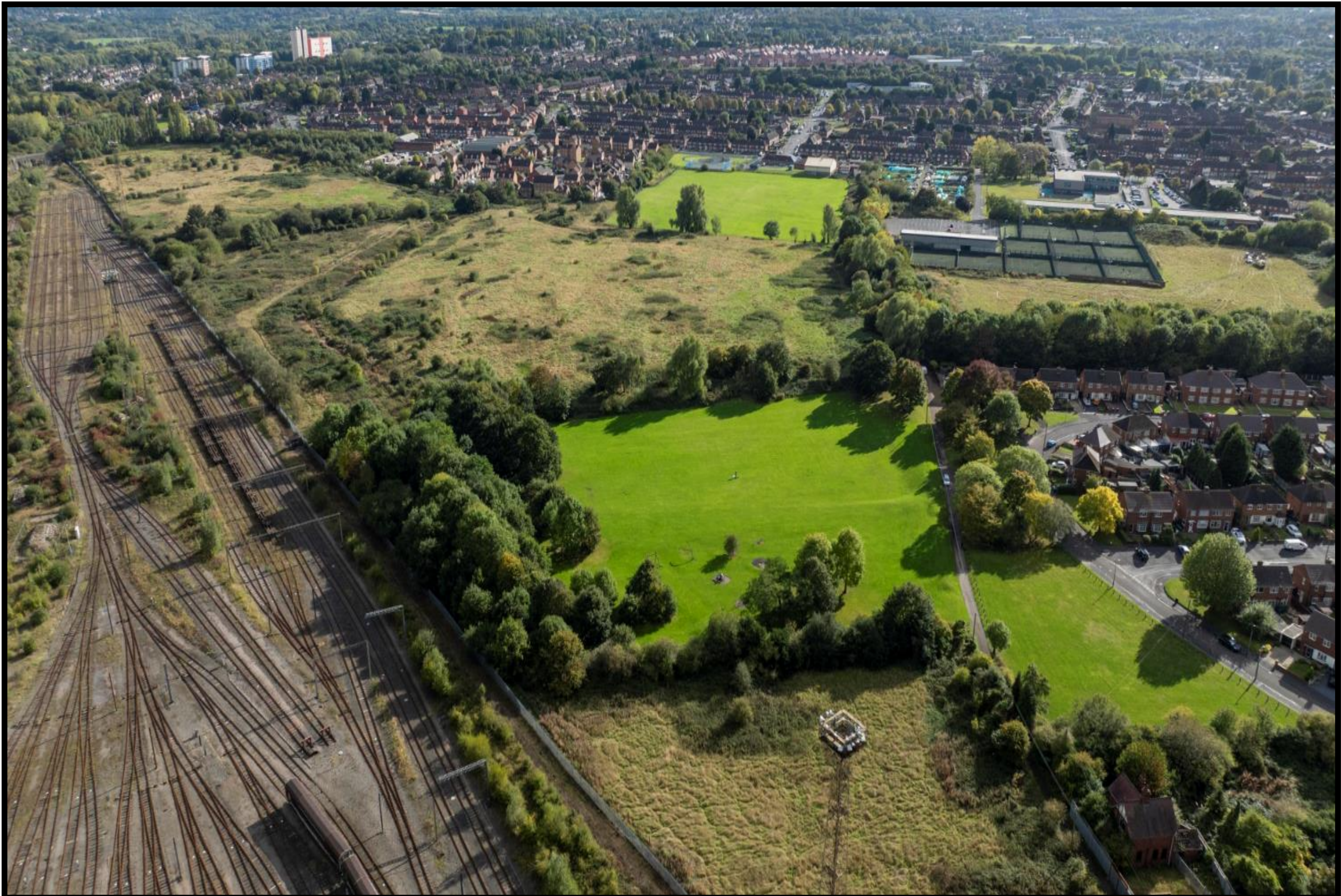
The Existing Site – Before the Proposed Remediation Works
